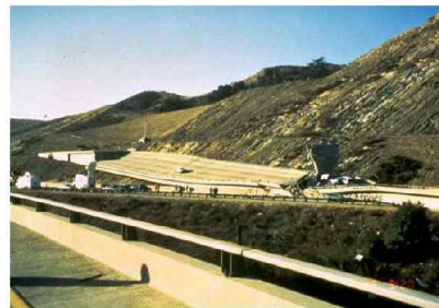
Bridge (West SR-14)
