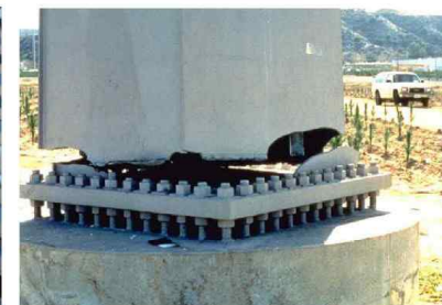
Electric Power Facility
